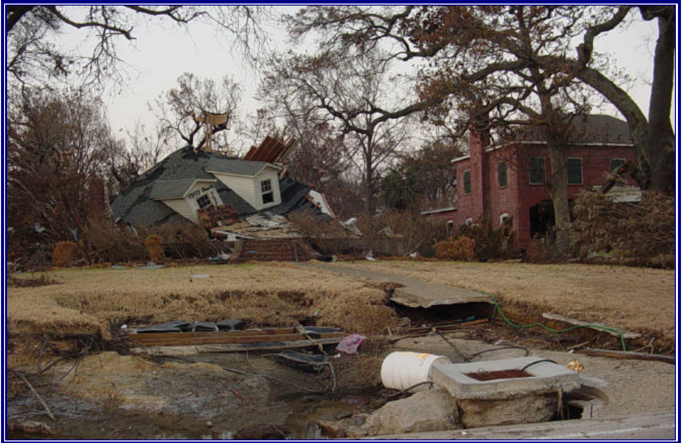
Damage caused by Katrina in Mississippi neighborhood.
