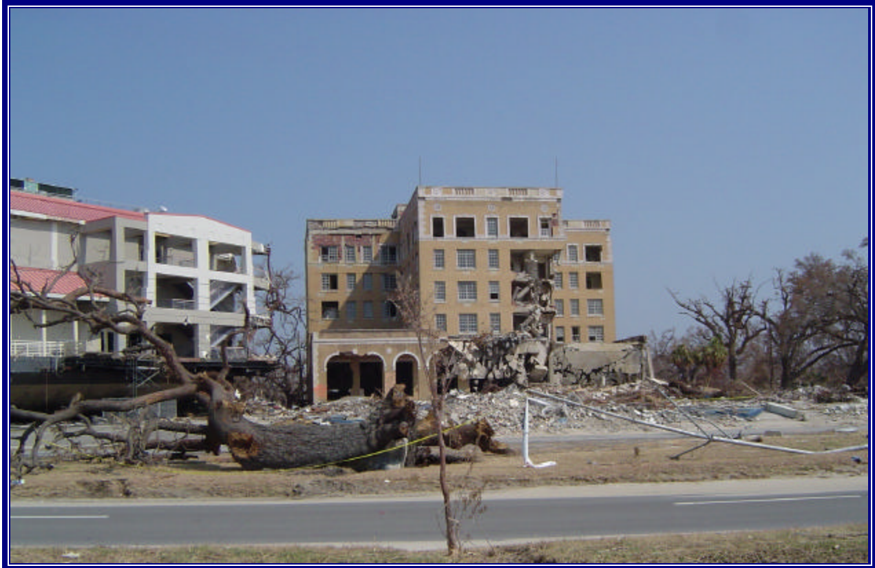
Damage caused by Katrina
