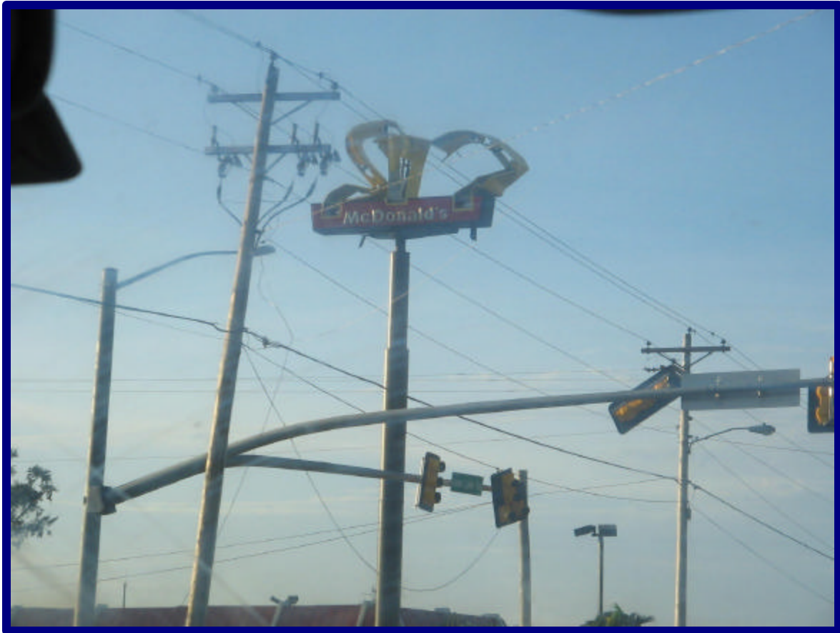
McDonald's sign damaged from Katrina
