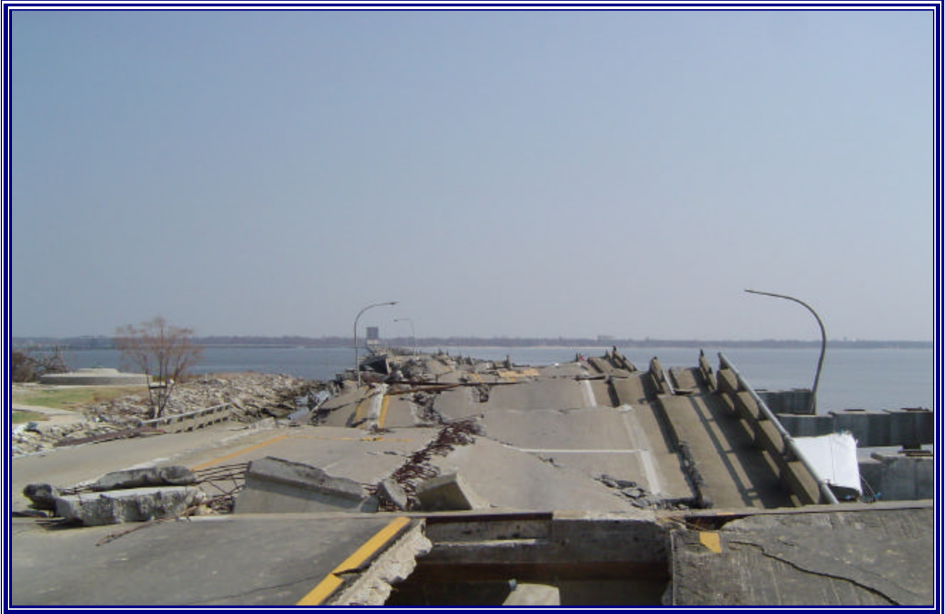
Road damage caused by Katrina
